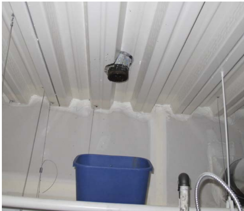
Existing drain pipe that was capped.
